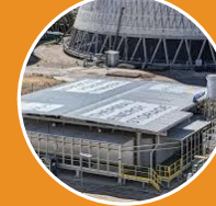
Thermal storage plants
